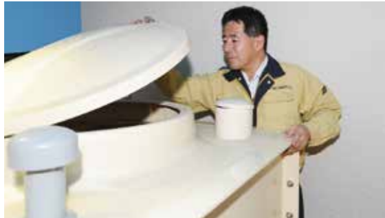
貯水槽の点検
